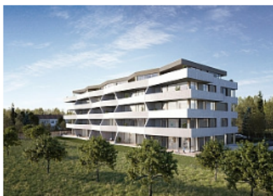
Leine Building, Paul-Flechsig-Straße 11
